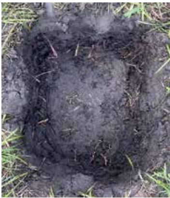
Figura 5: Hole dug to accept 8" fiber pedestal
