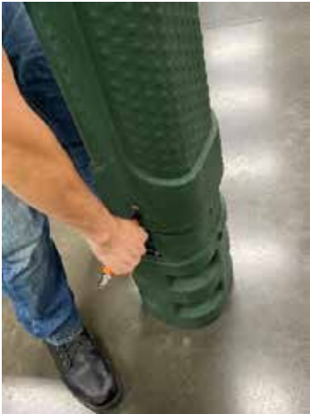
Figure 8: While maintaining the unlocked position, lift the lid of the fiber pedestal.
