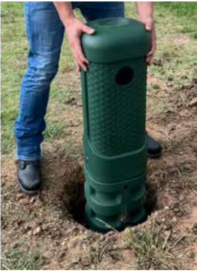
Figure 6: Lowering fiber pedestal into hole for installation.
