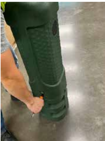
Figure 7: Unlocking fiber pedestal.
