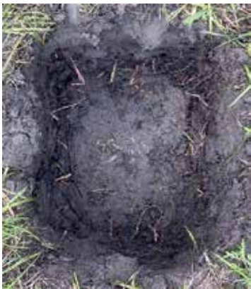
Figure 5: Hole dug to accept 8” fiber pedestal
