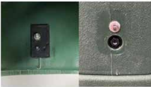
Figure 3: Location of self-locking mechanism on GOAT fiber pedestals is located on left side of pedestal unit.
