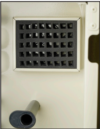
Unused splitter inputs/ outputs can be plugged into temporary panel for future expansion.
