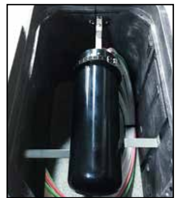
90° Splice closure mounting
