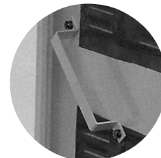
Above Ground Fiber Loop Storage Fastener
